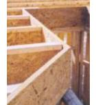
RIM BOARD PLUS is used where additional nail holding strength is siding or for attaching exterior deck ledger boards. RIM BOARD PLUS is a 1-1/8" thick OSB product. All RIM BOARD PLUS is APA stamped and edge sealed. Full units are wrapped to prevent weather damage. This product has an extremely high vertical design capacity at 5,700 lbs. per lineal foot.
